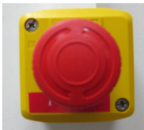
Figure 16. The emergency electrical shut down button may be a simple red button (A) and may be labeled with confusing wording such as “Emergency Stop” or “E Stop” (B).
