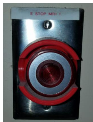
Figure 16. The emergency electrical shut down button may be a simple red button (A) and may be labeled with confusing wording such as “Emergency Stop” or “E Stop” (B).
