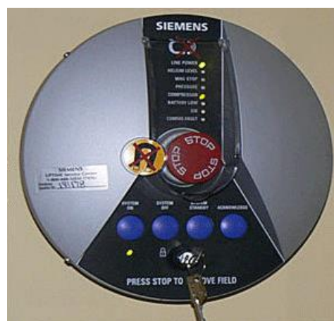
Figure 17. Sample quench buttons. (A) Plastic case must be opened and plastic cap removed to depress button. Quench will occur within 2 minutes. (B) Quench button labeled "STOP" under plastic lid secured by a "No Magnet" sticker. (From "Emergency shut...", 2017.)
